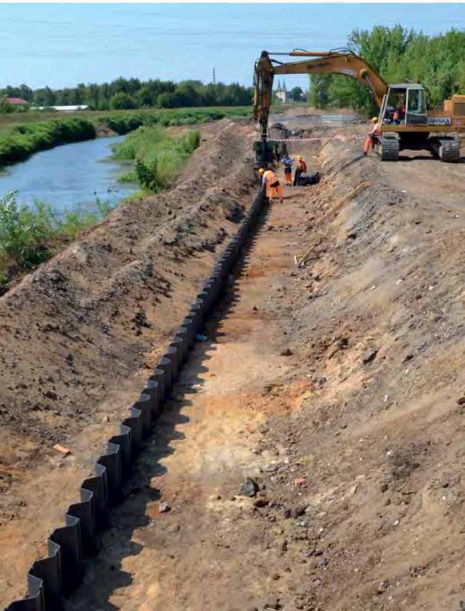
SCÈLÈMENT ET RENFORCEMENT DE LA DIGUE ANTI-INONDATION.
