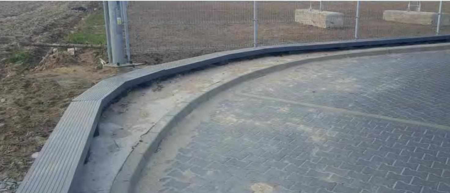
PROTECTION D'UNE STATION-SERVICE CONTRE INONDATION ET ORIENTATION DU CHEMIN DE FILTRATION DES EAUX AFIN D'AUGMENTER LA RÉTENTION DES ZONES AGRICOLES VOISINES. UNE STRUCTURE ÉTANCHE ASSURE UNE PROTECTION CONTRE LA CONTAMINATION CHIMIQUE.
