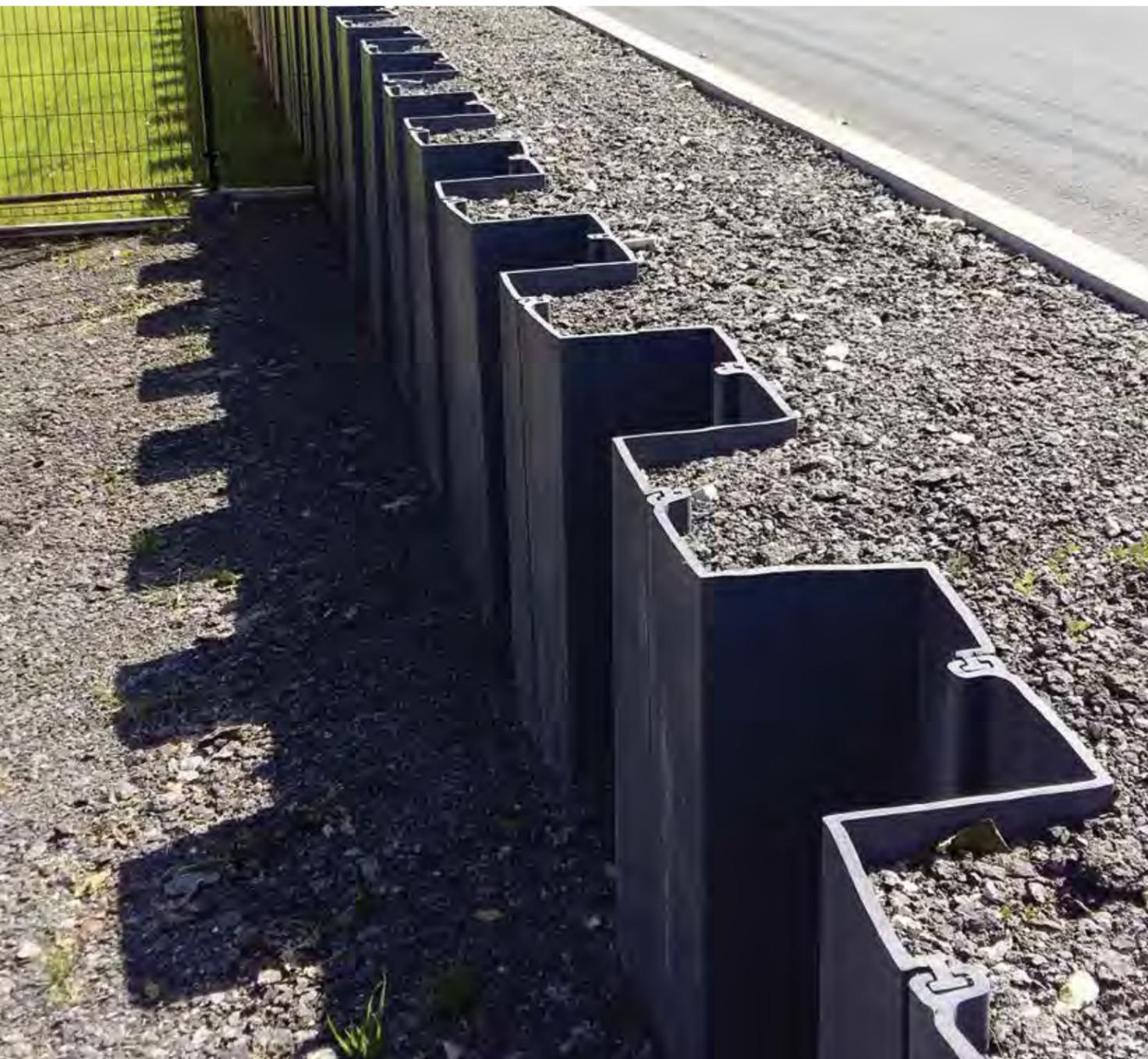
MUR DE SOUTÈNEMENT FAISANT L'ÉLÉMENT DE LA CONSTRUCTION DE ROUTE.
