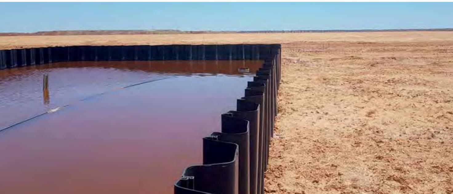
BASSIN D'EAU SALÉE RÉALISÉ EN PALPLANCHES EN VINYLE DOTÉES D'UN JOINT D'ÉTANCHÉITÉ INTÉGRALE EN PVC SOUPLE.
