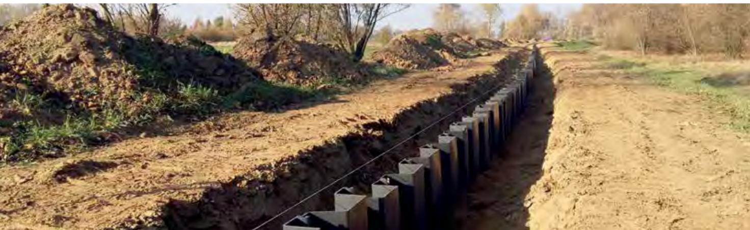
GIZAŁKI, POLOGNE: SCÉLLEMENT ET RENFORCEMENT DE LA DIGUE ANTI-INONDATION.
