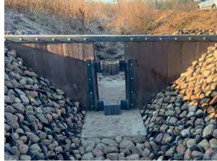
GRABÓW, POLOGNE: UN AUTRE TYPE DE BARRAGES DE RÉTENTION, INSTALLÉS DANS LA MÊME ZONE DE DRAINAGE DANS LE BASSIN DU FLEUVE PILICA.
