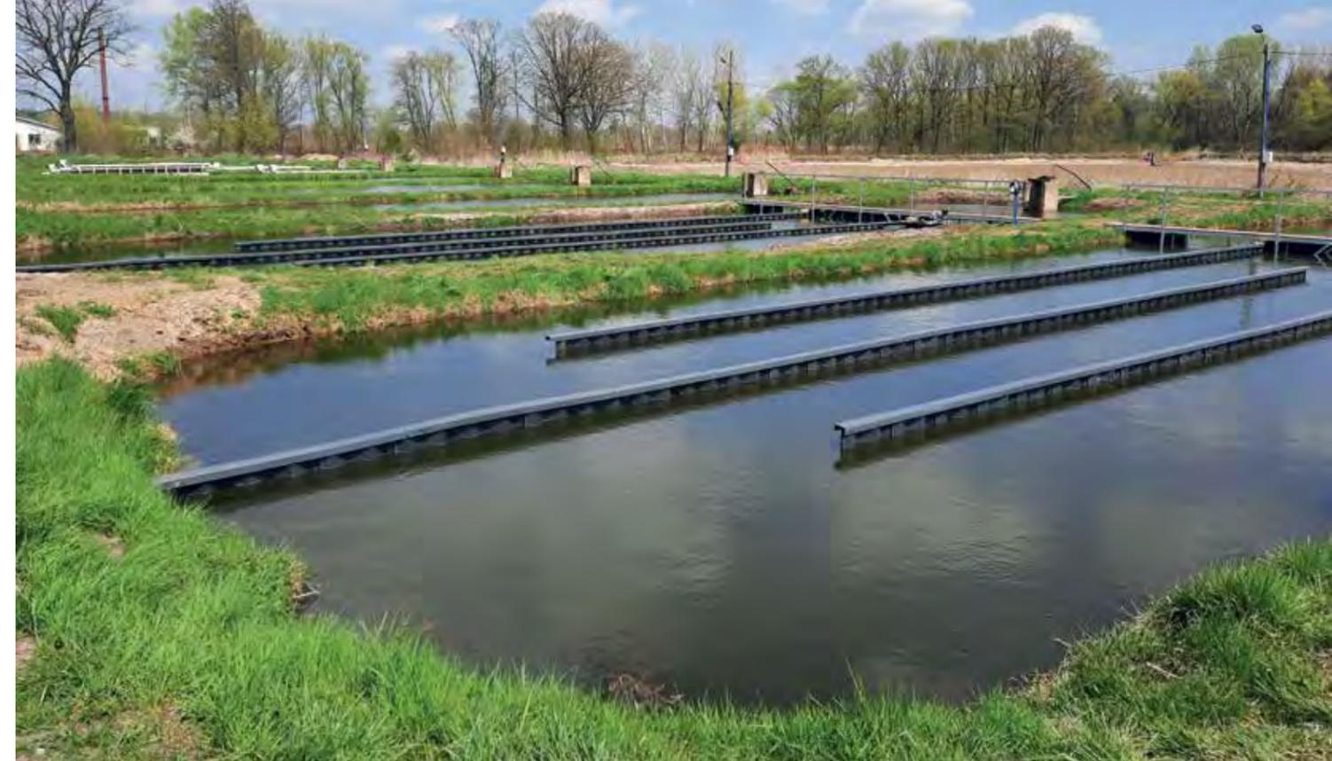
DES PALPLANCHES EN VINYLE ET DES PLANCHES TERRADECK UTILISÉES POUR LA CONSTRUCTION DE L'INFRASTRUCTURE AU SEIN DU COMPLEXE EXPÉRIMENTAL D'ÉTANGS DE PÊCHE DE ŻABIENIEC, POLOGNE.
