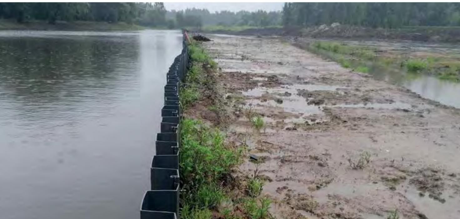
PALPLANCHES EN VINYLE DOTÉES D'UN JOINT D'ÉTANCHÉITÉ POUR UN DÉPLACEMENT TEMPORAIRE DU COURS D'EAU.
