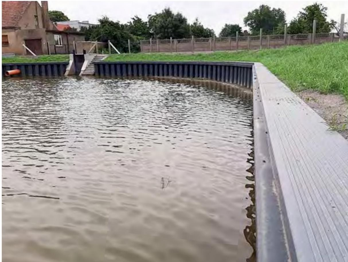
REVITALISATION DU BASSIN DE RÉTENTION - STABILISATION DES BERGES À L'AIDE D'UNE ENCEINTE EN PALPLANCHES EN VINYLE AVEC CAPUCHON ET MODERNISATION DE L'ÉVACUATION D'EAU PAR LA POSE D'UNE BARRAGE DE RÉTENTION DANS LE SEUIL EXISTANT.
