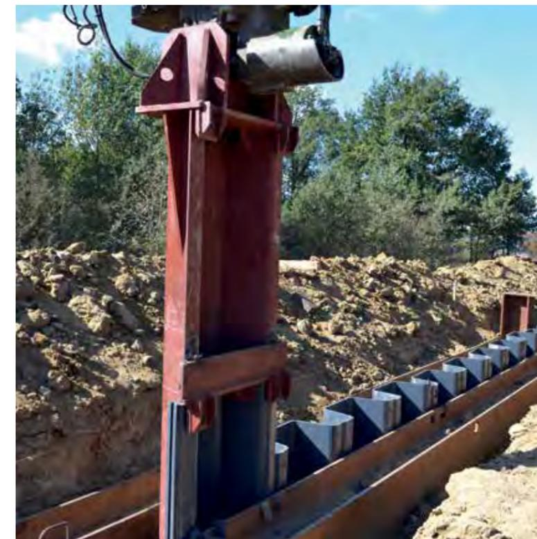
NOEUD DE TRANSPORT DE WROCLAW, POLOGNE: RENFORCEMENT D'UNE DIGUE ANTI-INONDATION PAR PALPLANCHES EN VINYLE - TRAVAUX D'INSTALLATION.
